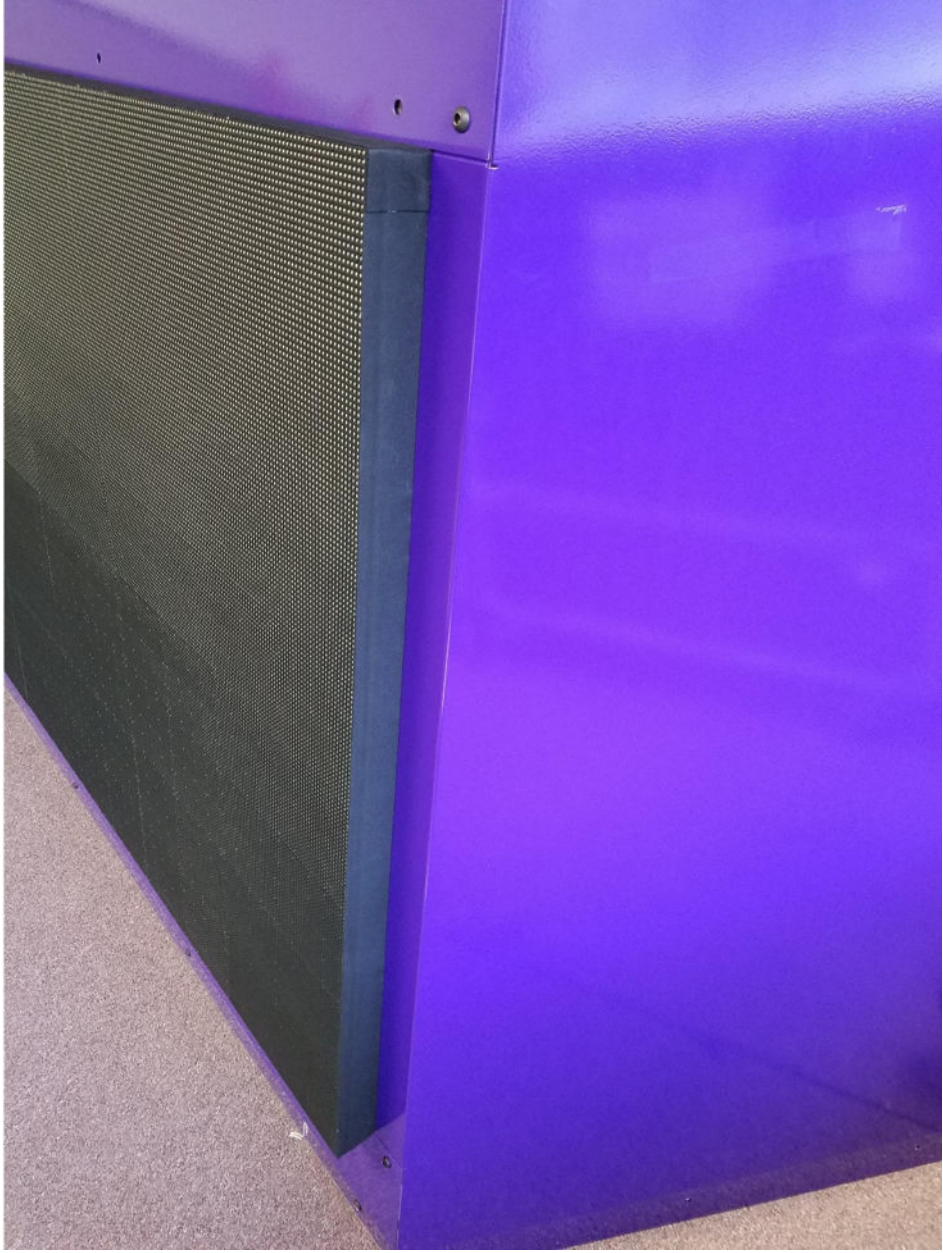
Install cover panels after foam tape is applied
